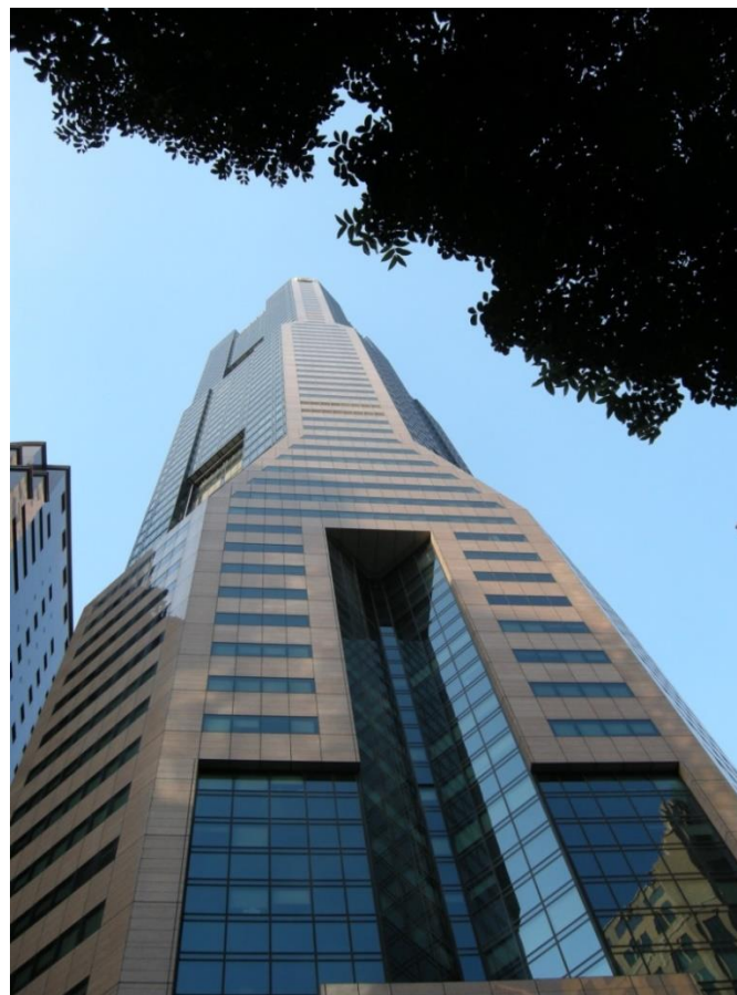
Singapore, Republic Plaza Building. (*3.2-5)
